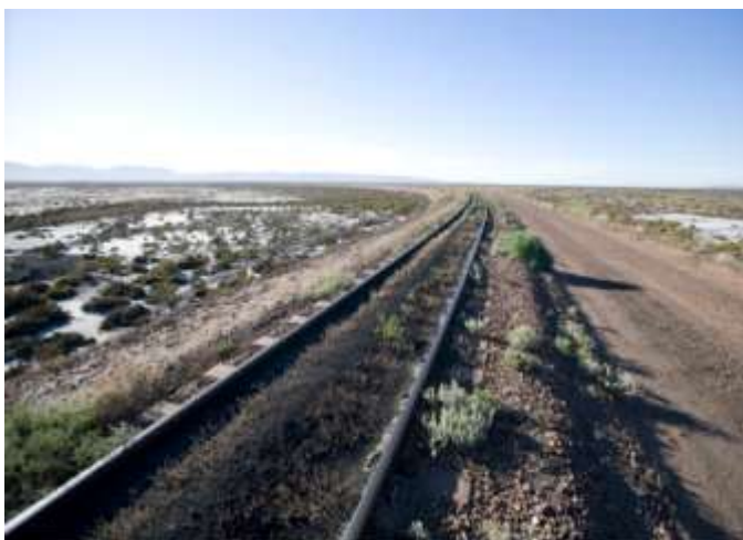
Existing Rail Loop
