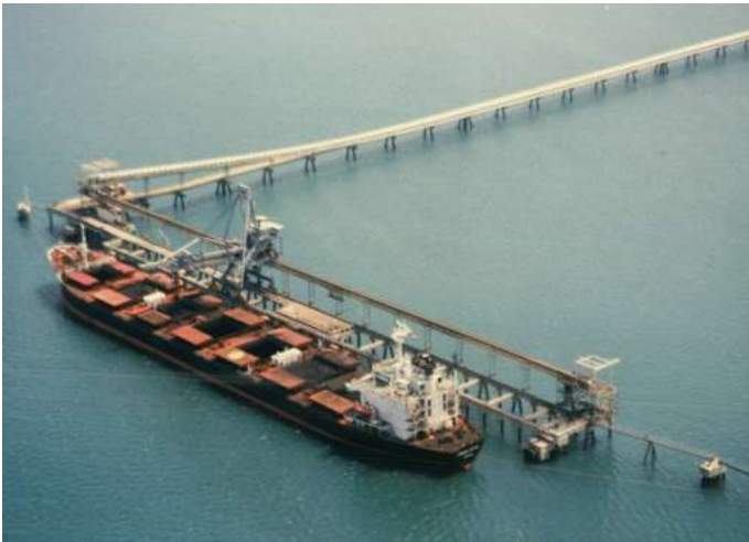
10Mtpa North Pulau Laut Coal Port Transshipment Facility
