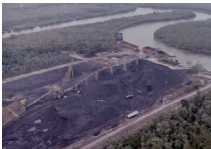
Satui, South Kalimantan Coal Port and Barge Load-Out Facility
