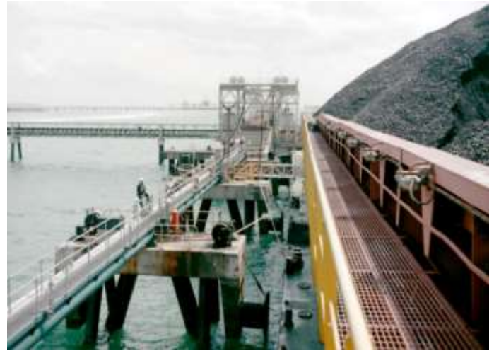
Barge Load In at NPLCT
