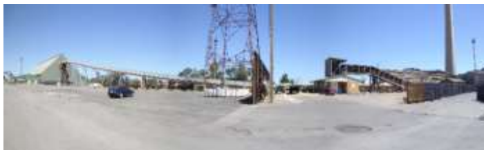
Berth Site, car located at Shiploader Pivot Point
