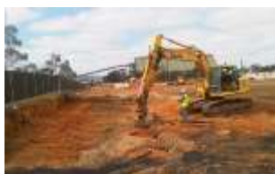
Bulk Earthworks at Storage Site
