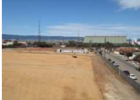
Transhipment Site following Site Earthworks
